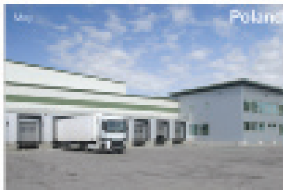
May Poland Builder: Skanska Budowlanych Customer: Zago Architect: DMAOO - Leszek Jank
