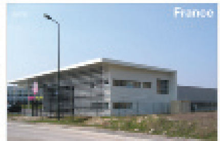
June France Builder: C.I.R. Customer: Impe/Buller Architect: BNA - Bernard Kinsler
