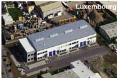
Builder: M.B.S. Buildings S.A. Customer: Ecostart II Architect: Paul Wurth
