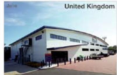
Builder: Mitchell Design & Construct Ltd Customer: Stamco Timber Ltd Architect: NA
