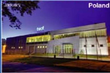
Builder: PW M. PASEK Sp. J. Customer: Best Poland Sp. o.o. Architect: Firma Inżynierska-Proceo
