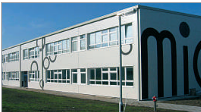
Builder: Moduling d.o.o., Slovenia Customer: Ministry of Education Architect: Jože Sraka
