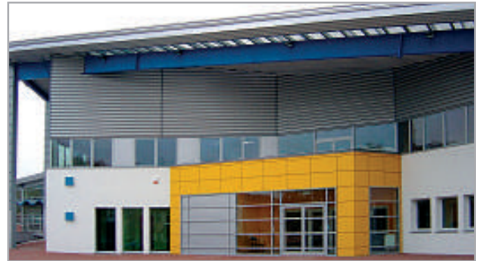
Builder: Asenhajmer Sp. z o.o., Poland Customer: Municipality Elblag Architect: Piotr Paldyna
